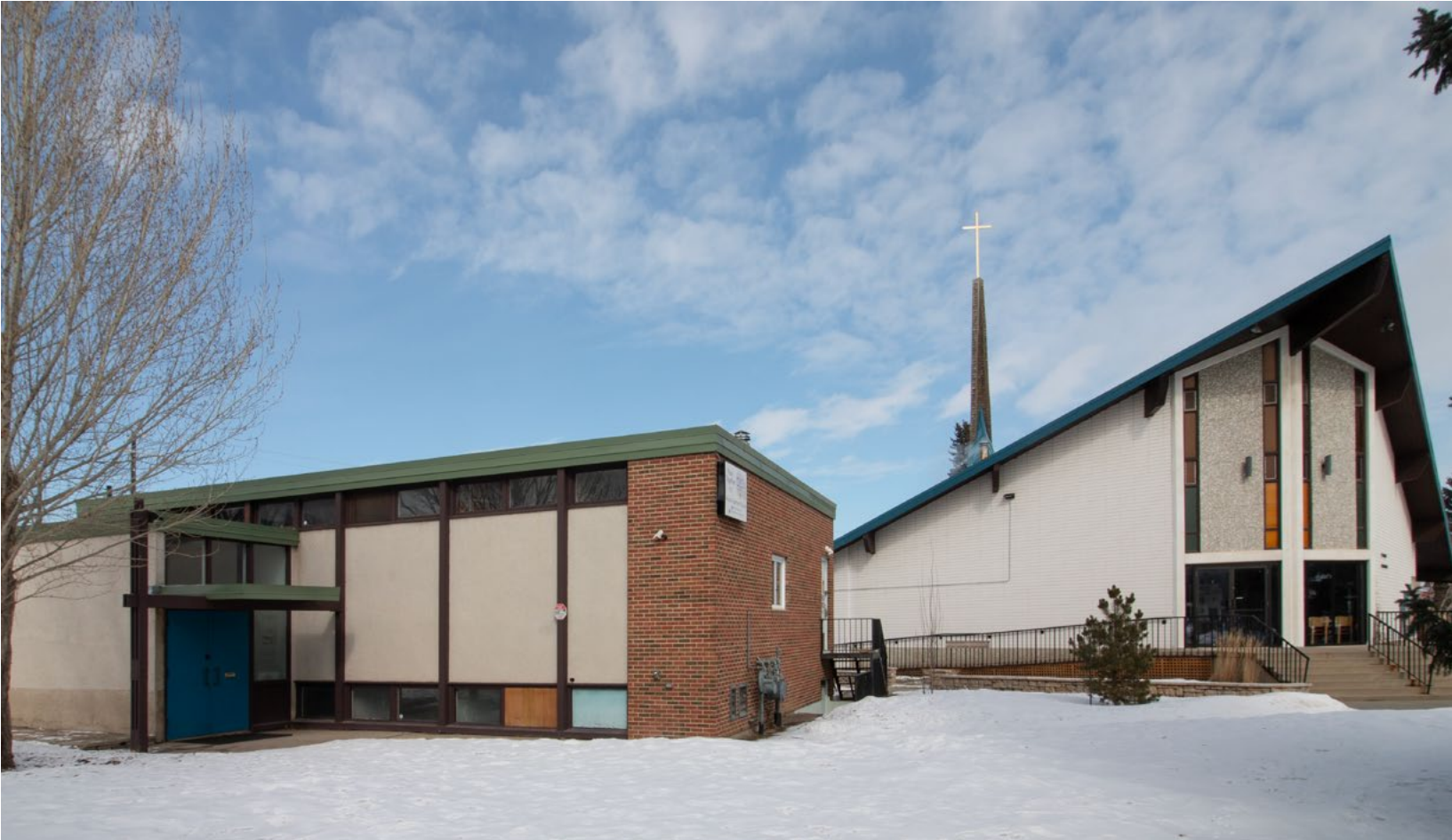
The St. Augustine’s Annex (left) and main building (right)
